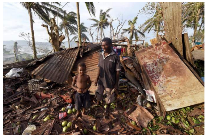
Devastation caused by Cyclone Pam - 2015
